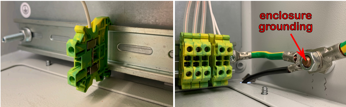
(a) Close-up view of a terminal block segment
