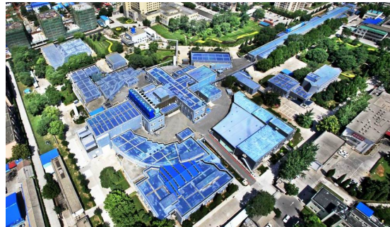
(b) Picture of BEPCII buildings [Ins18].
