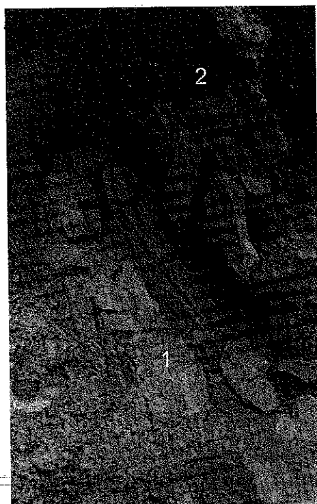
Fig.6 Märkisches Sauerland. Detail of blast furnace Nr. 1 (1 opened drainage; 2 hole for the bellows).
