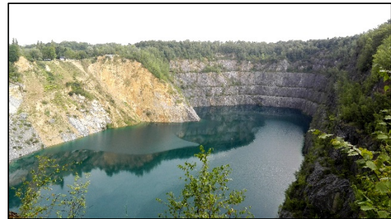
Fig. 8. The hardly studied, now lake-filled, well-bedded middle Givetian reef limestone quarry north of the Neanderthal Valley. The quarry wall collapse to the right ended most of the active operations.
