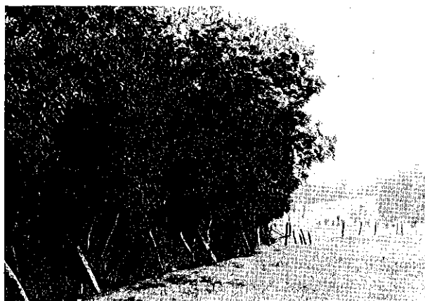
Fig. 6 Wooded slope of a hollow lane. There is a competition between element and grasland for light, water and nutrition. Fence is in a bad condition. Clearing of the maintenance arear increases the chance of preservation of the element.
