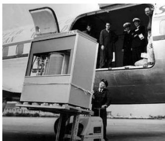
Photo: A 5MB IBM hard drive being loaded
