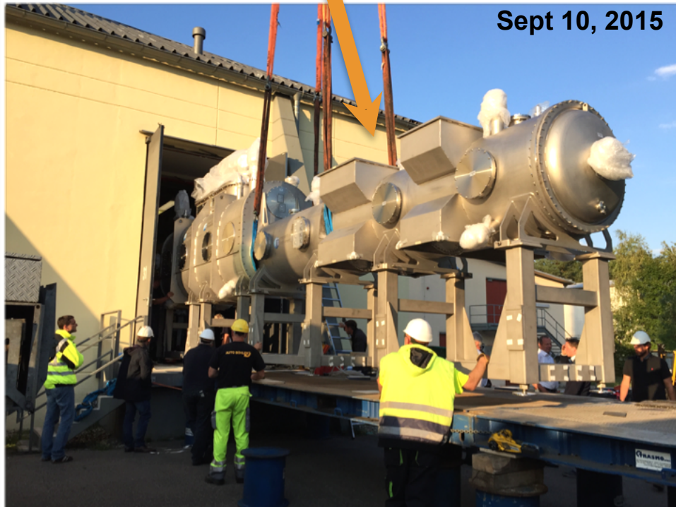
windowless gaseous tritium source
